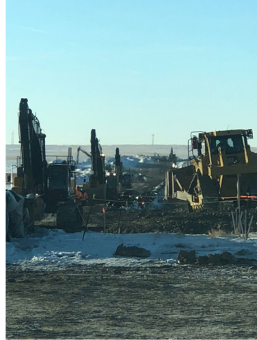
20. Backfill - km170+700 – Feb 9, 2018
