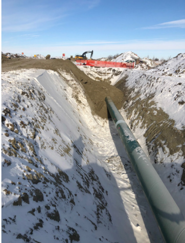
13. Backfill – Km 168+990 – Feb 7, 2018
