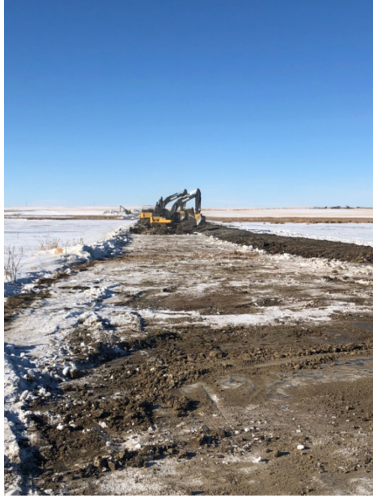
25. Clean up crew at wetland crossing – Feb 10, 2018
