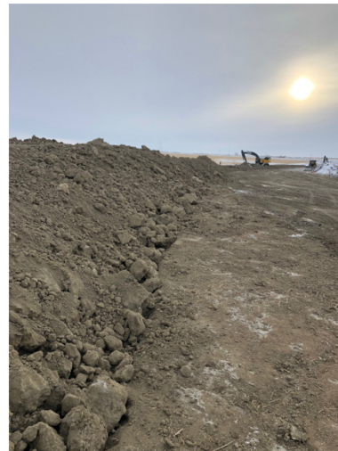
18. Backfilled mainline - km166+700 – Feb 8, 2018
