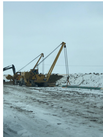
4. Tie-in - Km 166+600 – Feb 5, 2018
