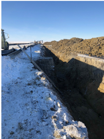
7. Backfill tie-in – Km 164+500 – Feb 6, 2018
