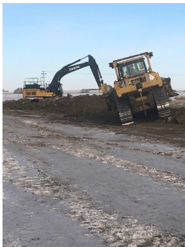
11. Dozer and excavator clean up– Km 166+650 – Feb 7, 2018
