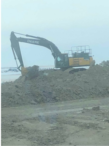
19. Excavator clean up - km168+800 – Feb 8, 2018
