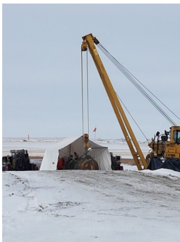
5. Welding pull head – Km 170+750 – Feb 5, 2018
