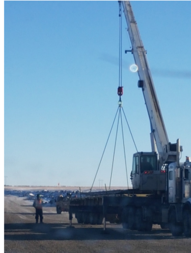
22. Loading mat – Km 166+700 – Feb 9, 2018
