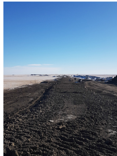
24. Backfilled tie-in – km 169+450 – Feb 10, 2018
