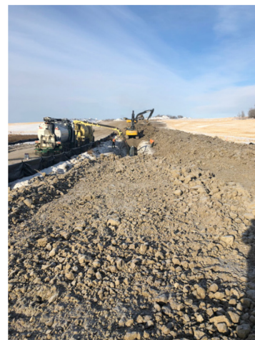
12. Excavator and hydrovac – km 164+600 – Feb 7, 2018
