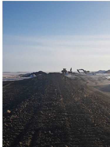
16. Backfill tie-in – km 168+850 – Feb 8, 2018
