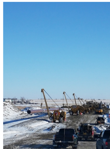
6. Lowering in (Wetlands)– Km 170+000 – Feb 6, 2018
