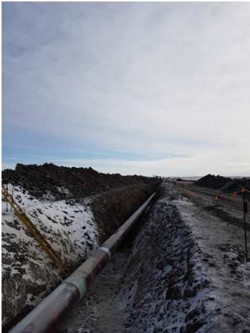
15. Shading pipe - km 170+200 – Feb 7, 2018
