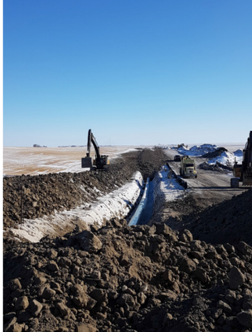
7. Backfill tie-in – Km 164+500 – Feb 6, 2018
