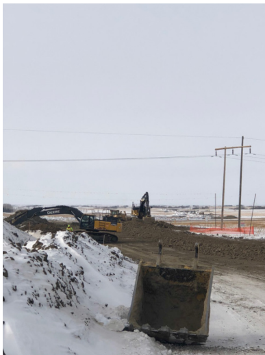
17. Excavator and dozer -167+750 - Feb 8, 2018
