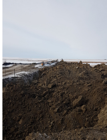
14. Shaded ditch - Km 170+750 – Feb 7, 2018
