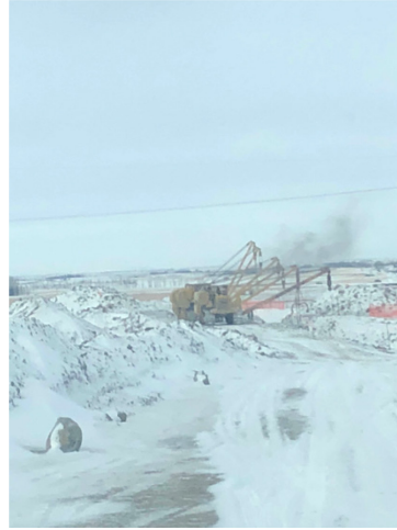
2. Booms going under power line – SF 98 – Feb 5, 2018
