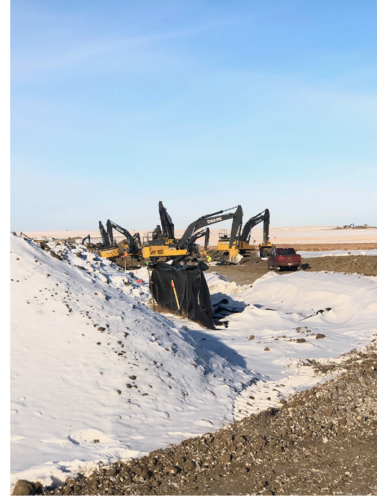
26. Clean up crew – km 170+650 – Feb 10, 2018
