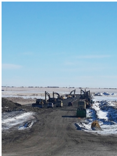
23. Equipment on wetland – km 169+950 – Feb 10, 2018
